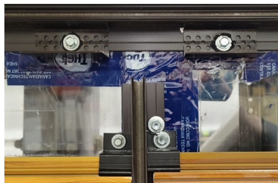
Photo No. 13 Fastener locations at mid-span
