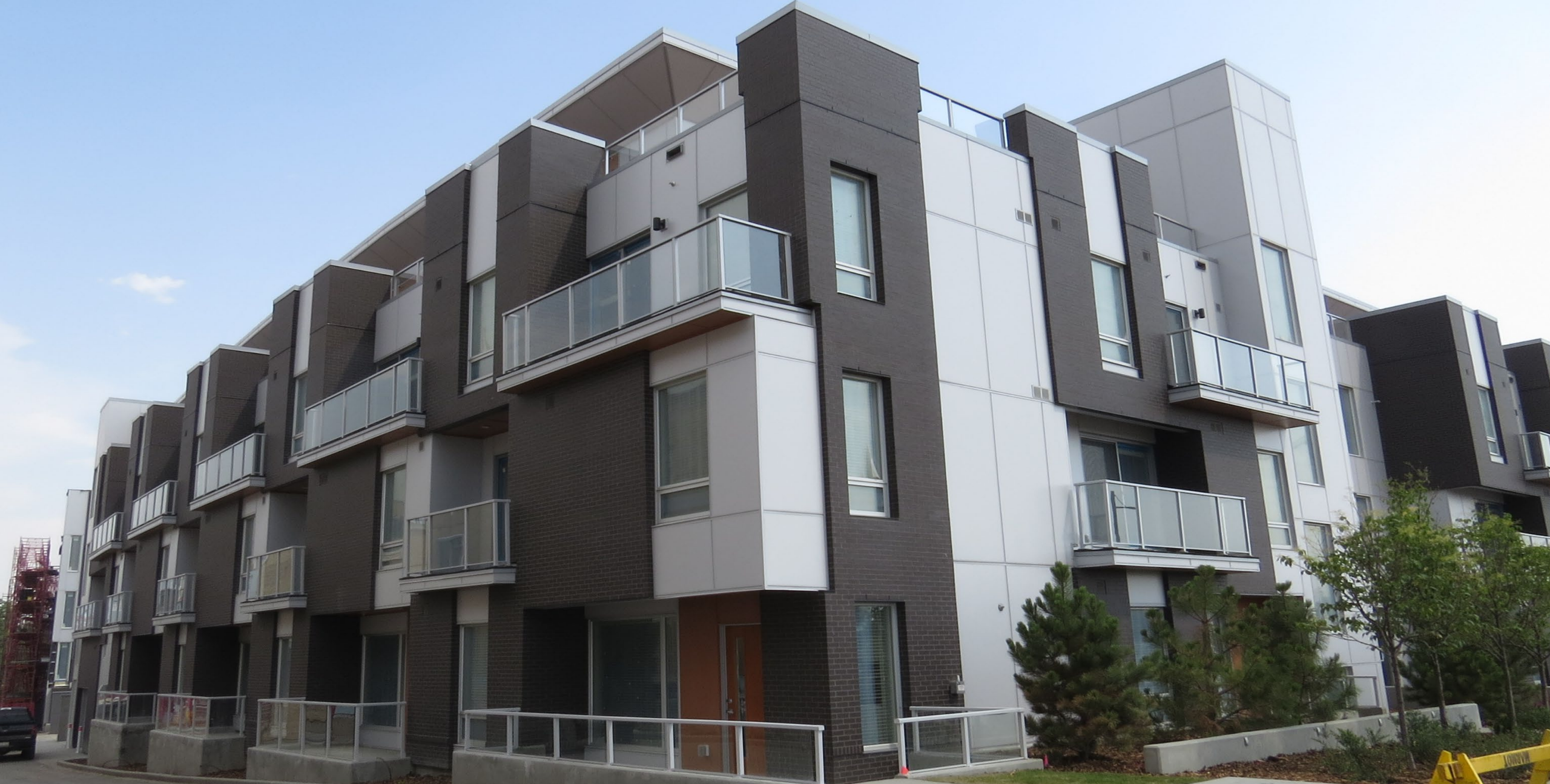
PROJECT: West Campus, University of Calgary | LOCATION: Calgary, Canada | COLOR: Palladium (custom color) with matching trims
