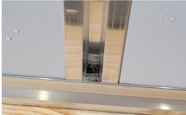
Photo No. 7 Vertical joint at sill
