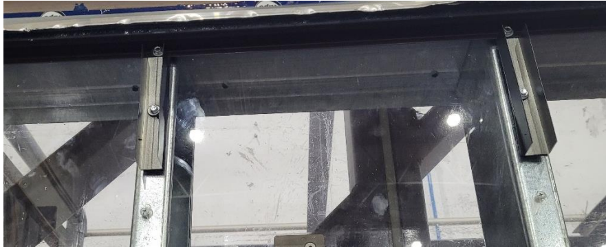
Photo No. 11 Spacer profiles at top of system
