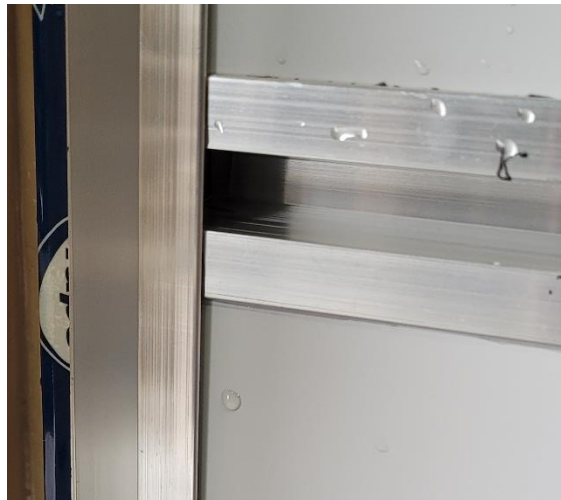
Photo No. 5 Horizontal joint at jamb
