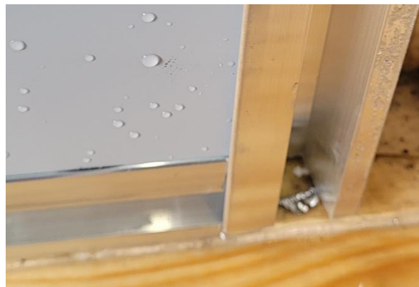
Photo No. 6 Jamb connection at sill
