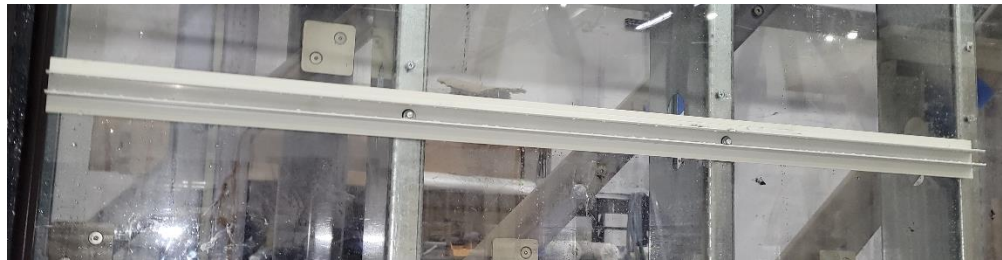
Photo No. 8 Stiffener track secured to wall
