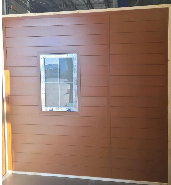
Photo No. 1 Test assembly – Exterior
