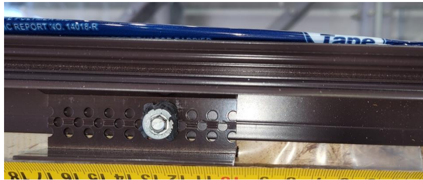
Photo No. 9 Top installation track
