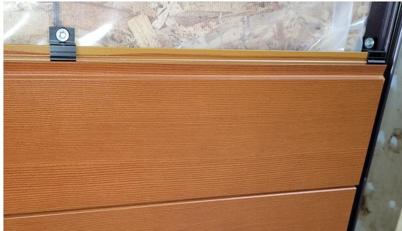
Photo No. 10 Installation clips
